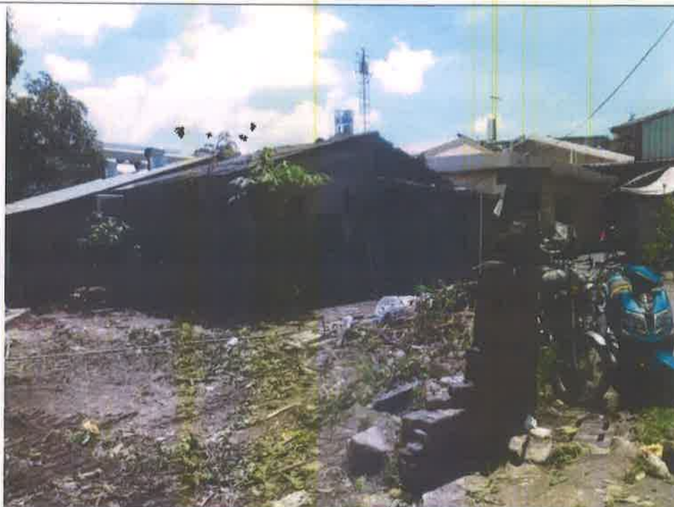
施工後照片2 Photos after construction2
