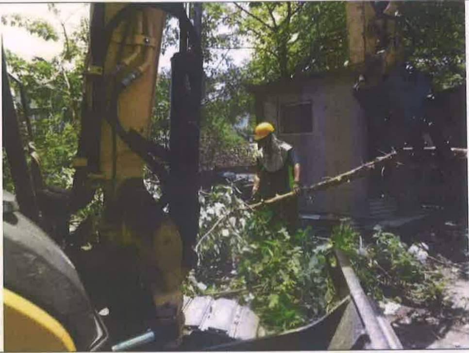
施工中照片1 Photos during construction1
