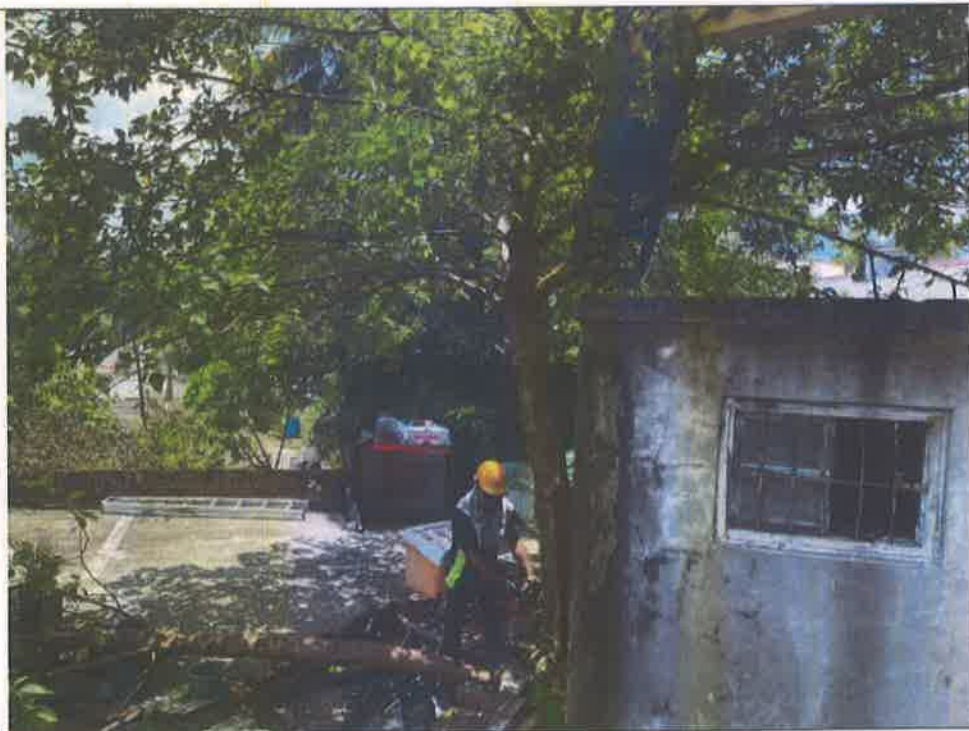
施工中照片2 Photos during construction2
