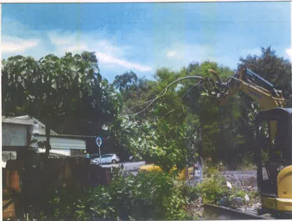
施工中照片2 Photos during construction2
