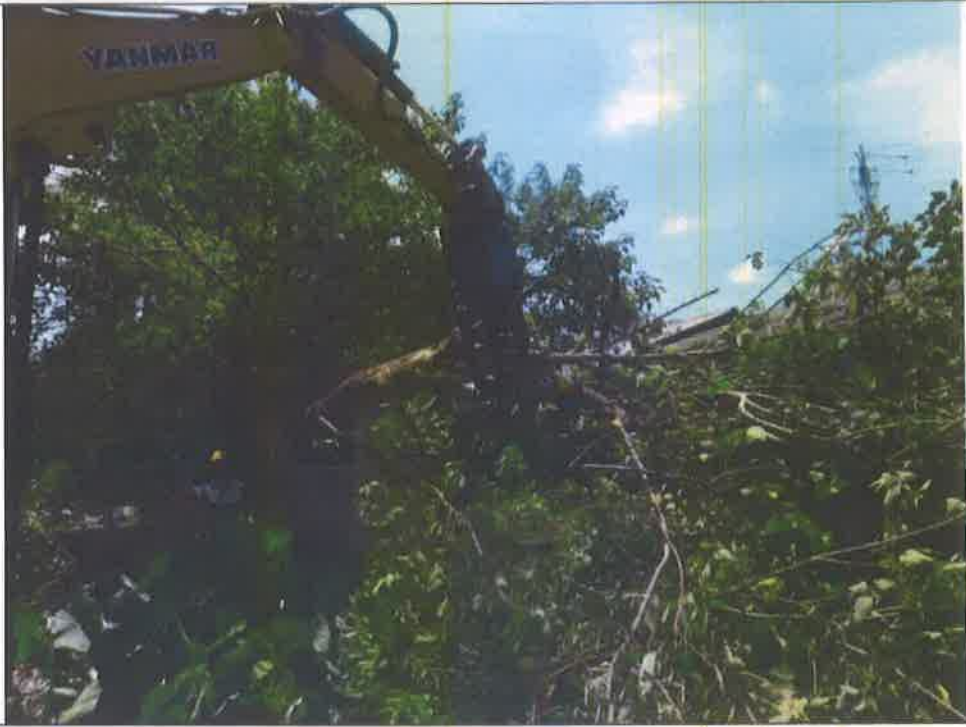
施工中照片1 Photos during construction1
