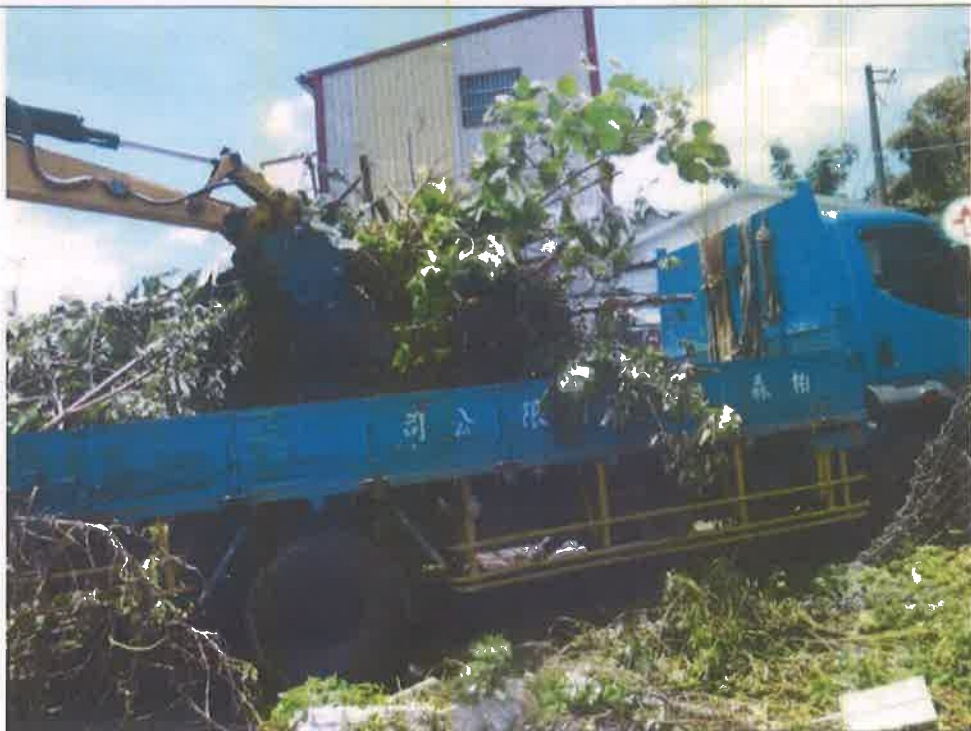
施工中照片2 Photos during construction2
