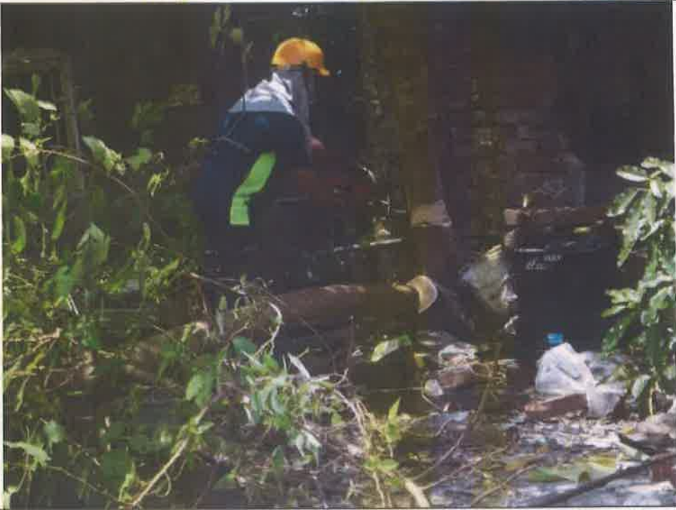
施工中照片1 Photos during construction1
