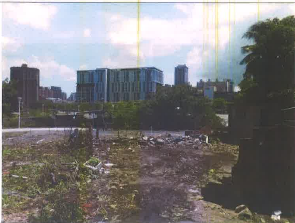
施工後照片1 Photos after construction1
