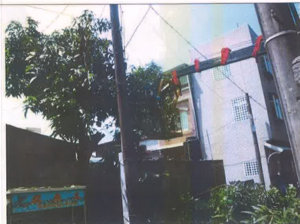
施工中照片2 Photos during construction2
