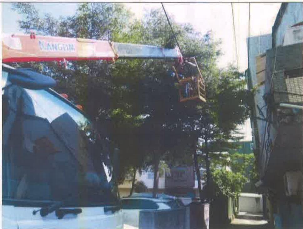
施工中照片2 Photos during construction2
