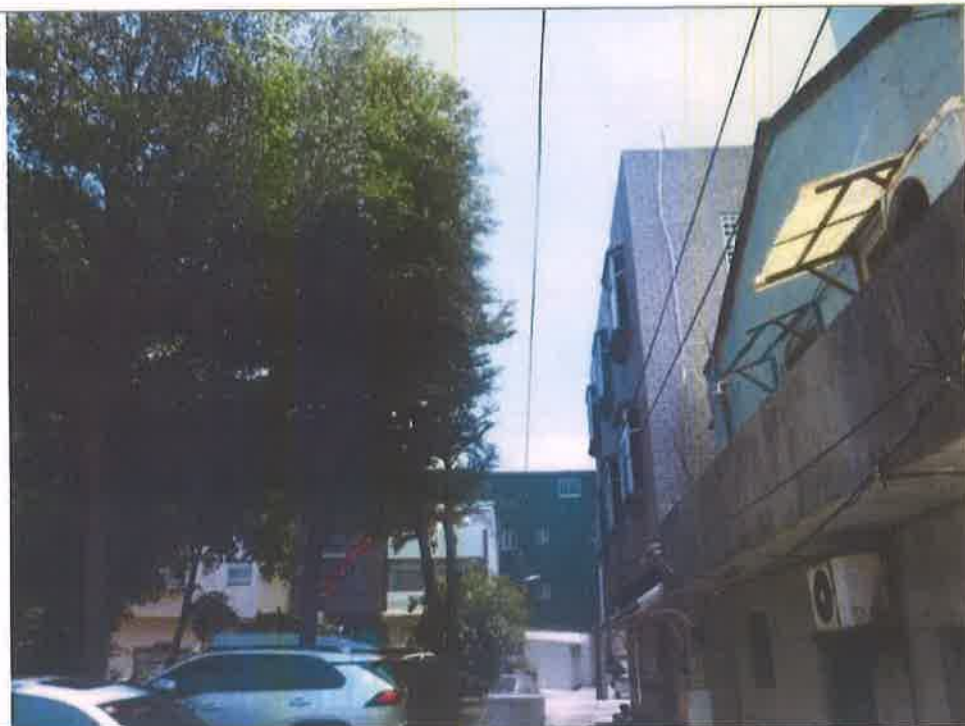
施工後照片1 Photos after construction1
