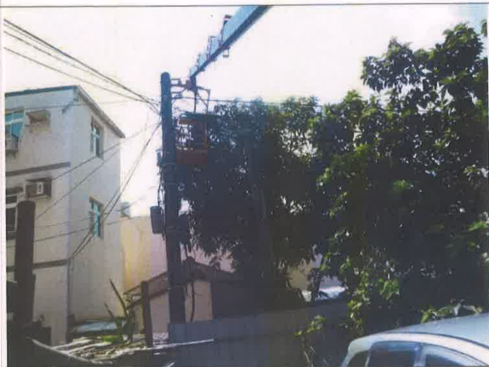
施工中照片1 Photos during construction1
