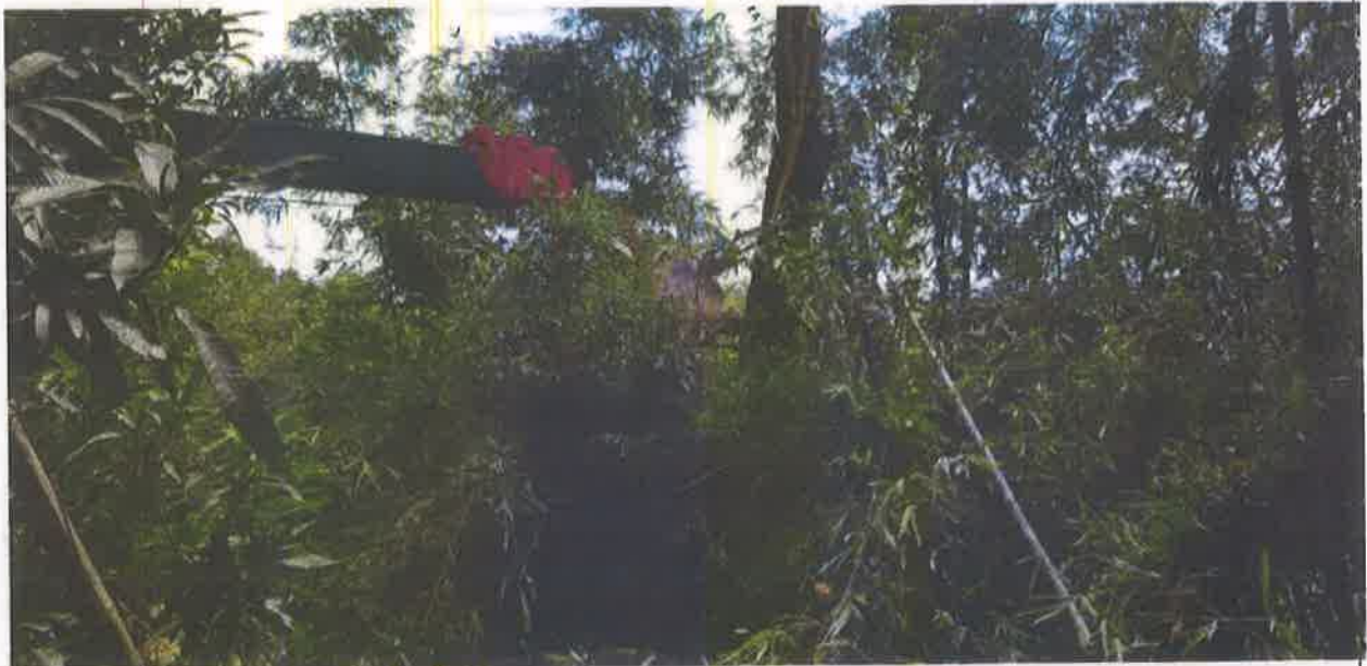
施工中照片2 Photos during construction2
