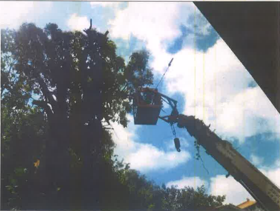
施工中照片2 Photos during construction2
