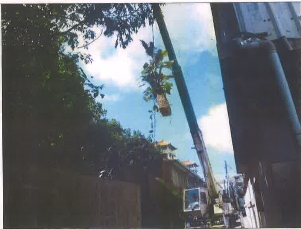
Photos during construction2
