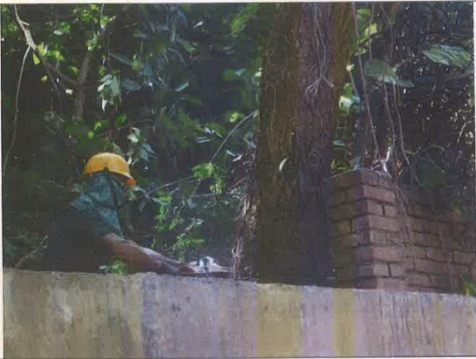
Photos during construction1
