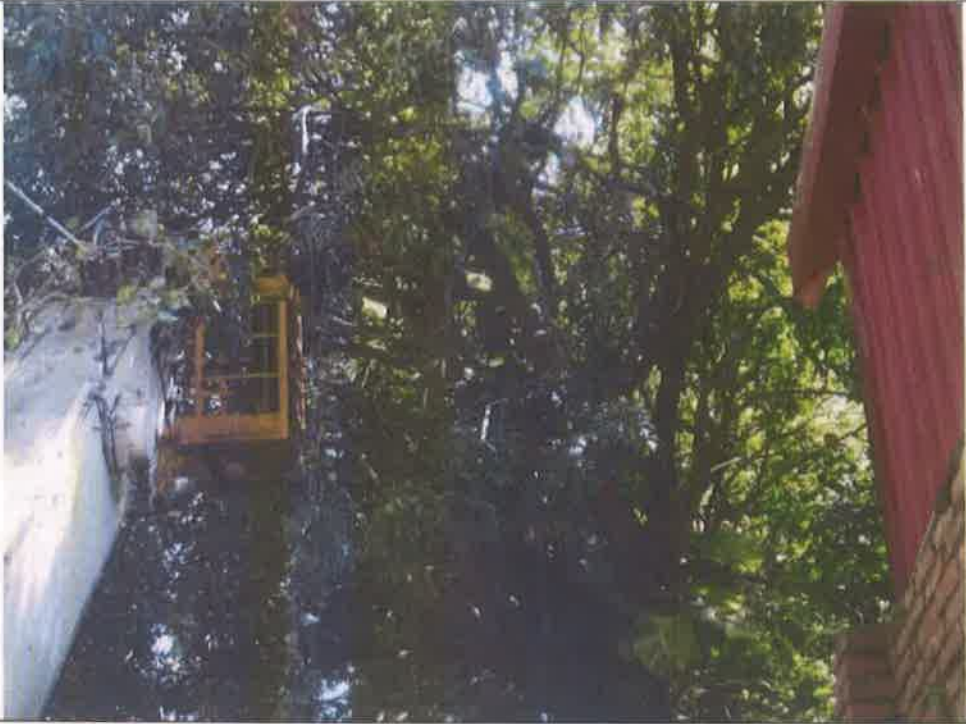
施工中照片1 Photos during construction1
