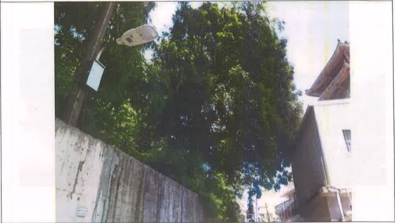
施工前照片1 Photos before construction1
