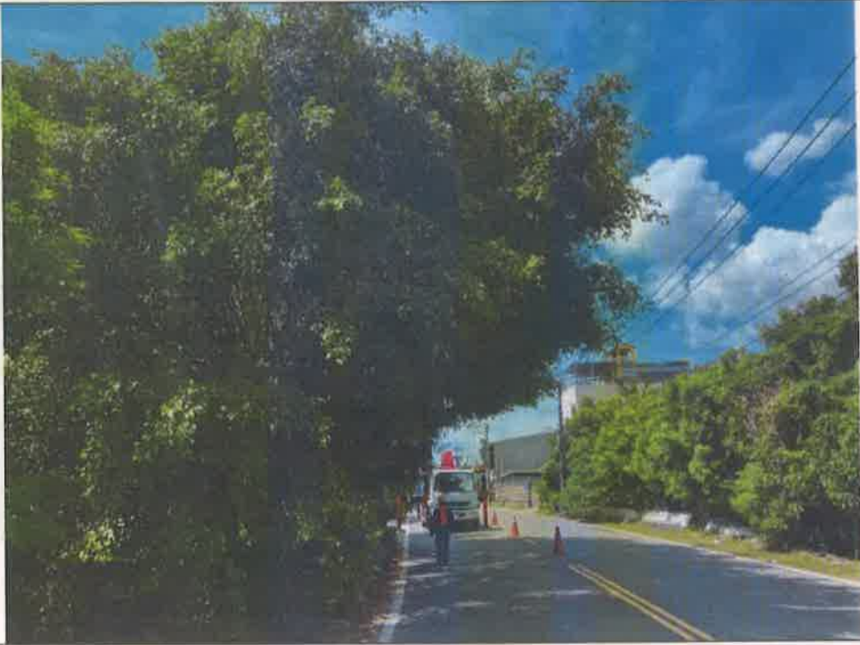
施工前照片1 Photos before construction1
