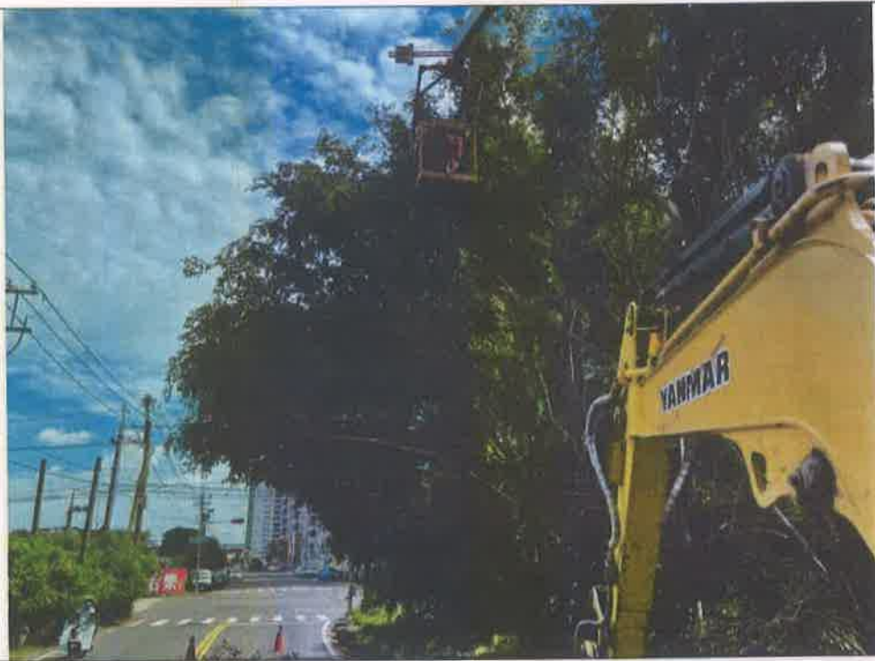
施工中照片2 Photos during construction2
