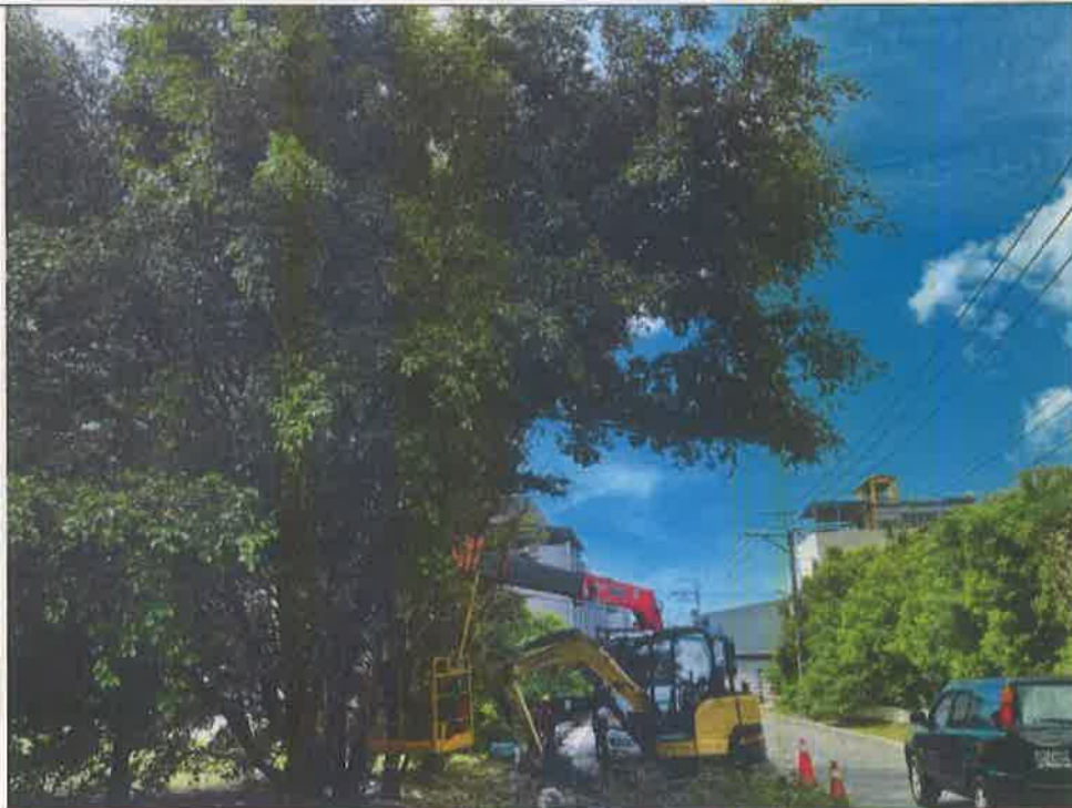
施工中照片2 Photos during construction2
