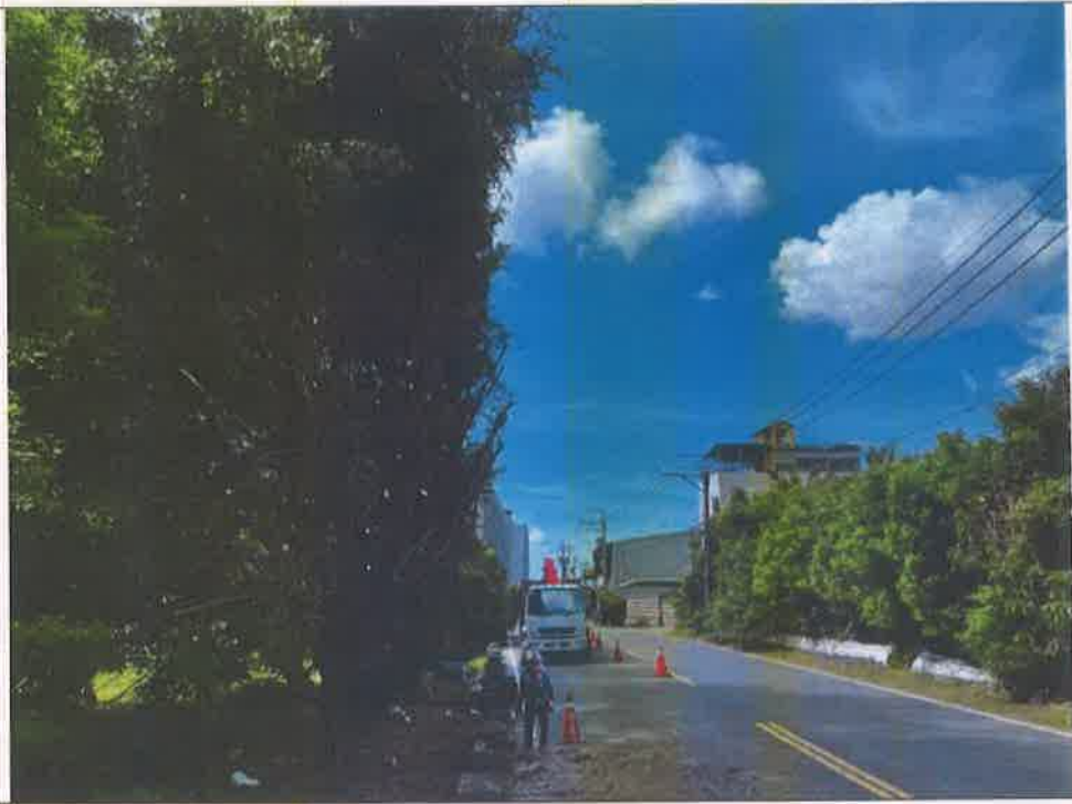
施工後照片1 Photos after construction1
