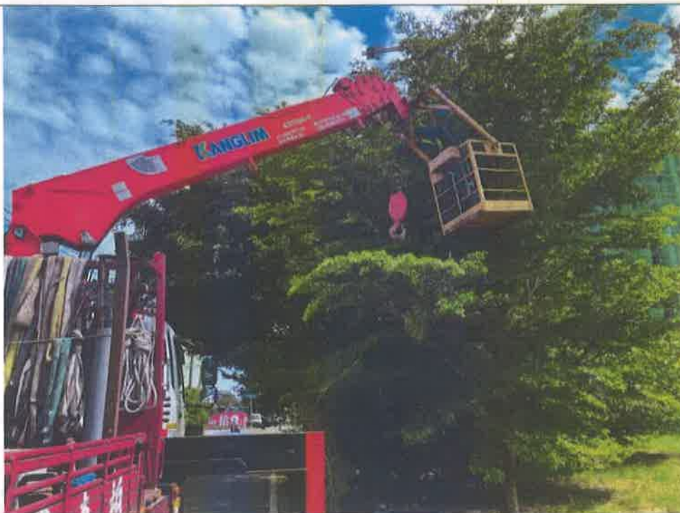
施工中照片1 Photos during construction1
