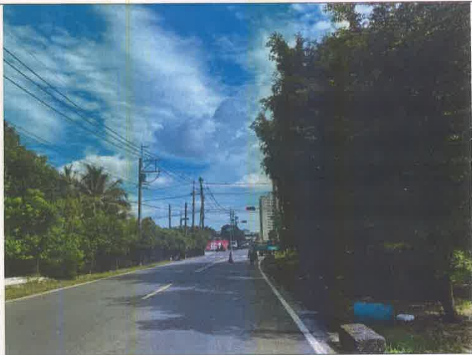
施工後照片2 Photos after construction2
