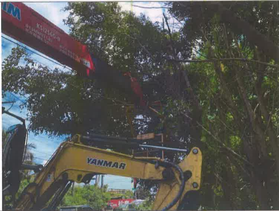
施工中照片1 Photos during construction1
