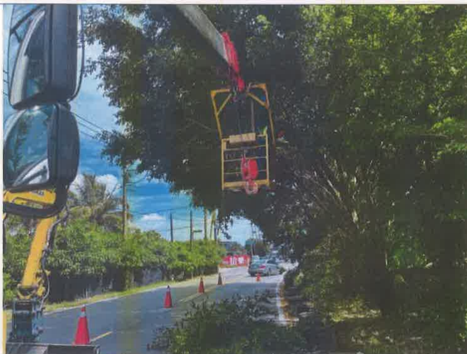
施工中照片2 Photos during construction2
