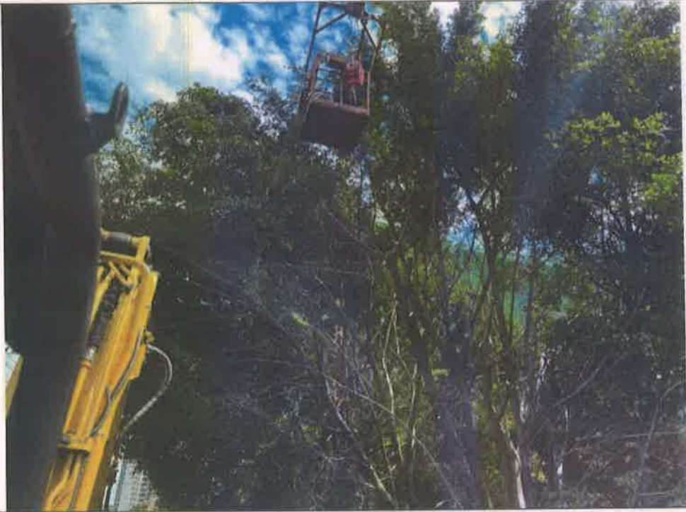
施工中照片1 Photos during construction1
