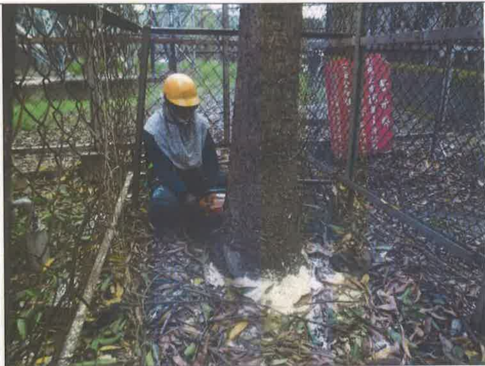
施工中照片2 Photos during construction2
