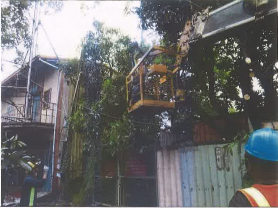
施工中照片1 Photos during construction1
