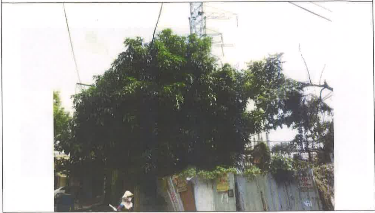
施工前照片1 Photos before construction1
