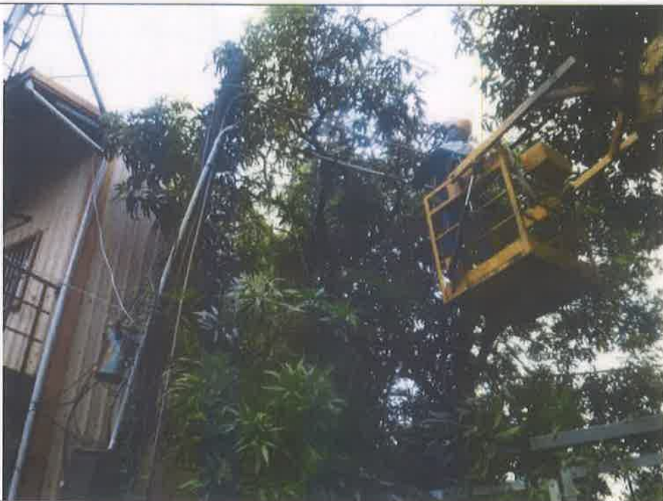
施工中照片2 Photos during construction2
