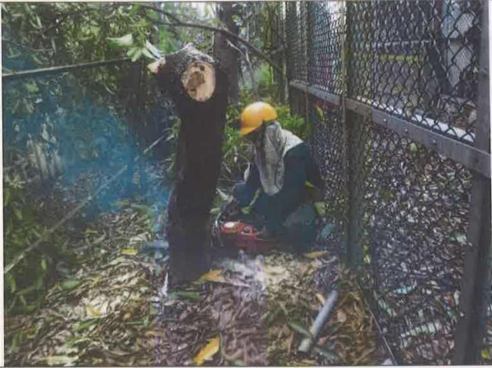
施工中照片1 Photos during construction1
