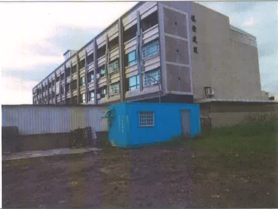
施工後照片1 Photos before construction1
