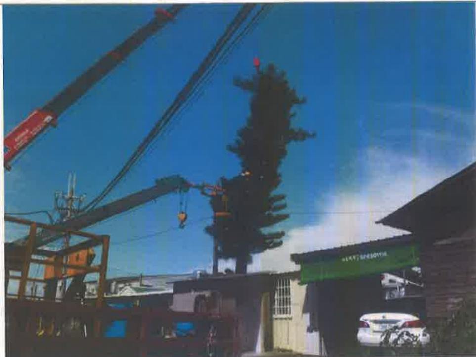
施工中照片1 Photos during construction1
