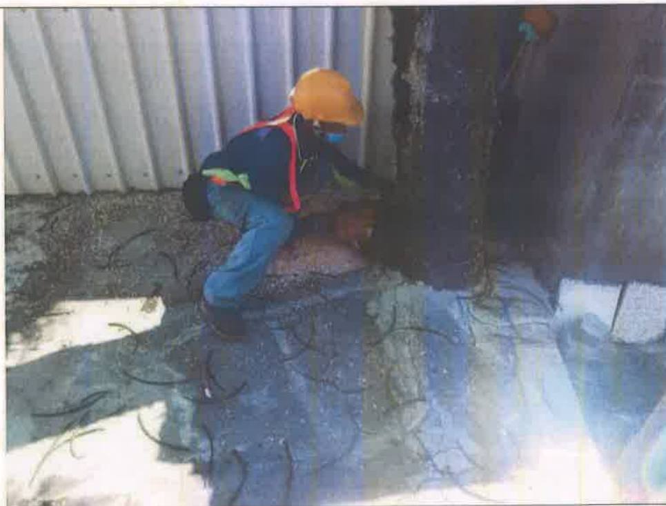
施工中照片2 Photos during construction2
