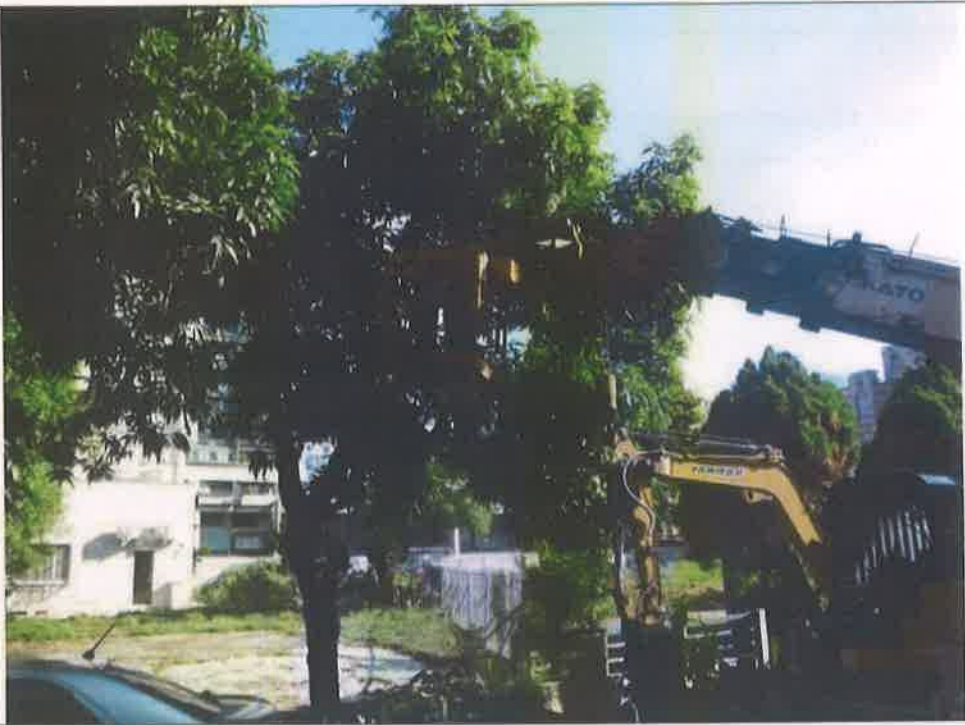
Photos during construction1
