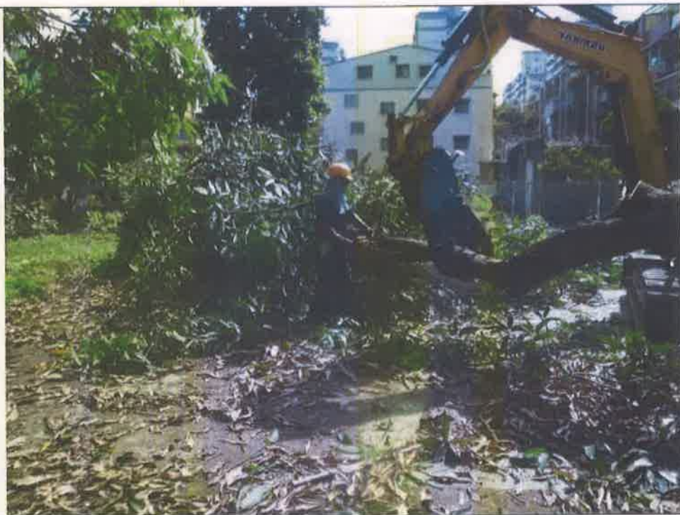
施工中照片2 Photos during construction2
