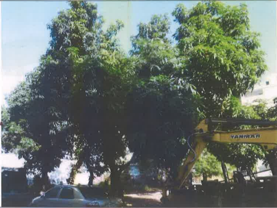
施工前照片1 Photos before construction1
