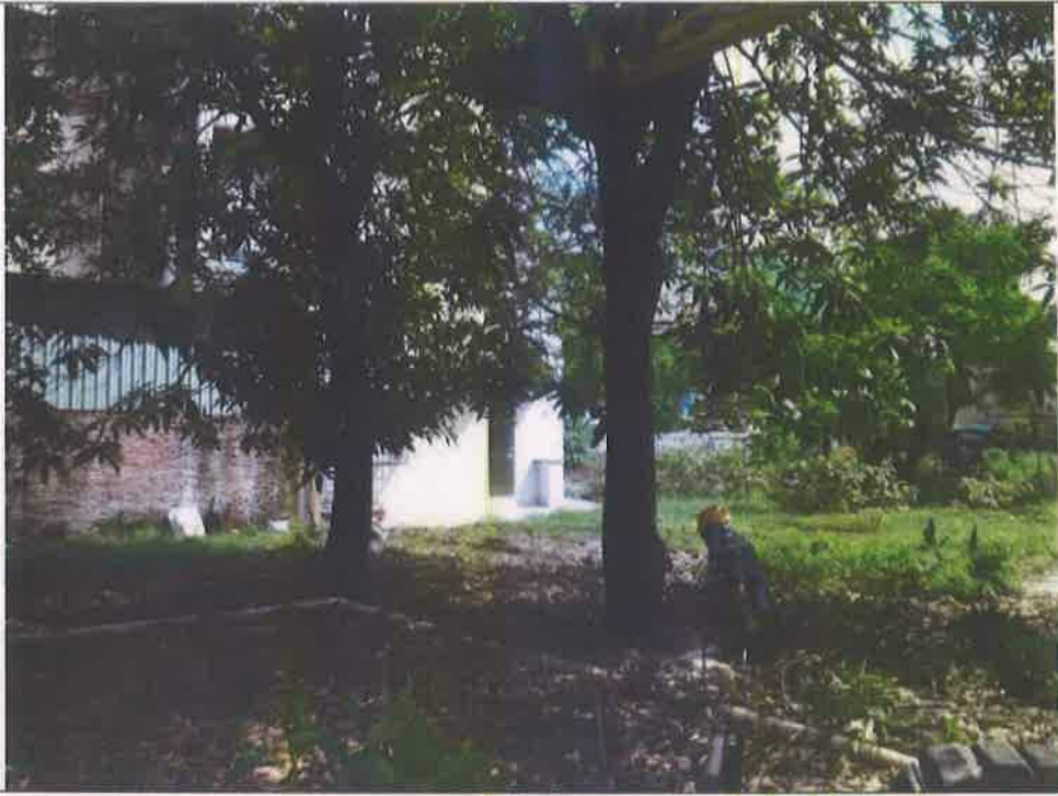
施工中照片1 Photos during construction1
