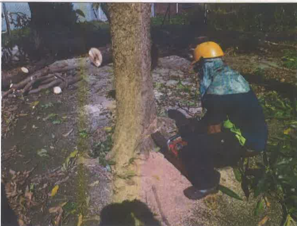
施工中照片2 Photos during construction2
