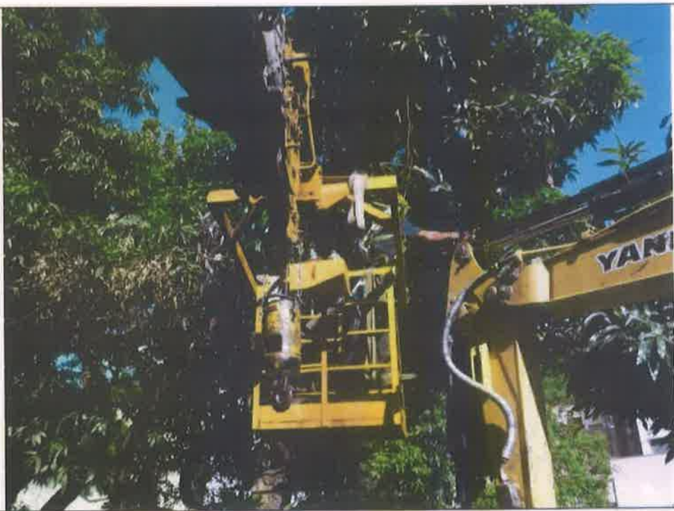
Photos during construction2
