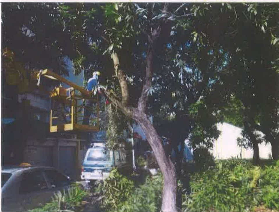
施工中照片1 Photos during construction1
