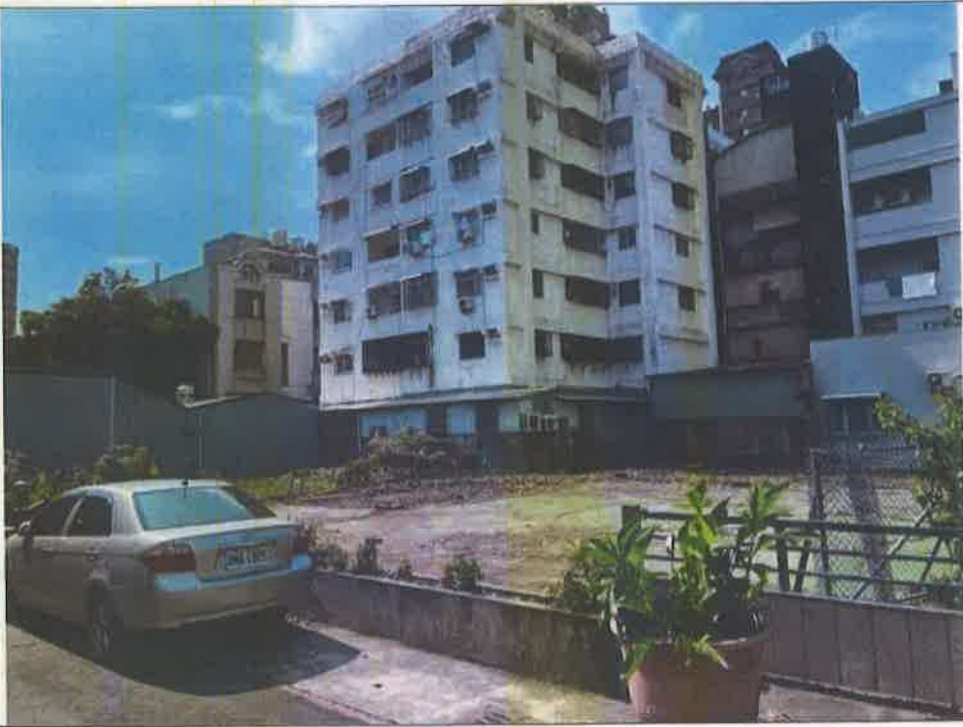
施工後照片1 Photos after construction1
