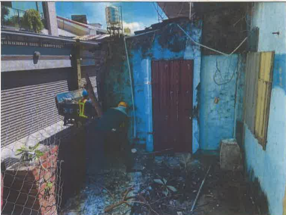
施工中照片2 Photos during construction2
