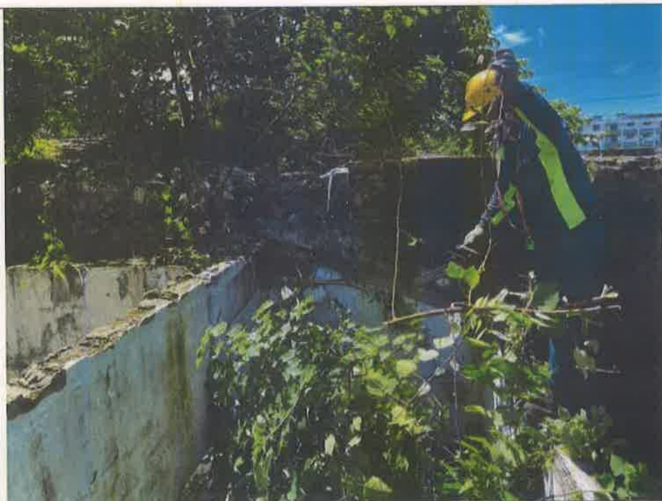
施工中照片2 Photos during construction2
