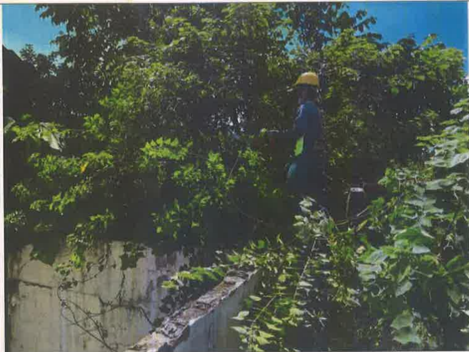
施工中照片1 Photos during construction1
