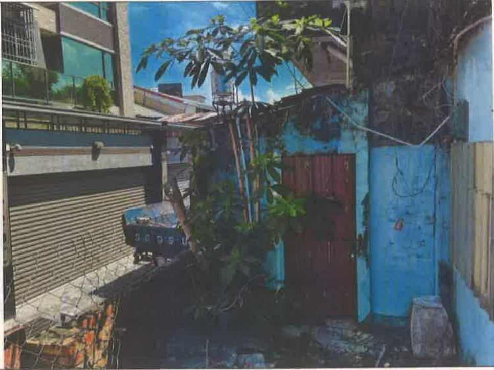
施工前照片1 Photos before construction1
