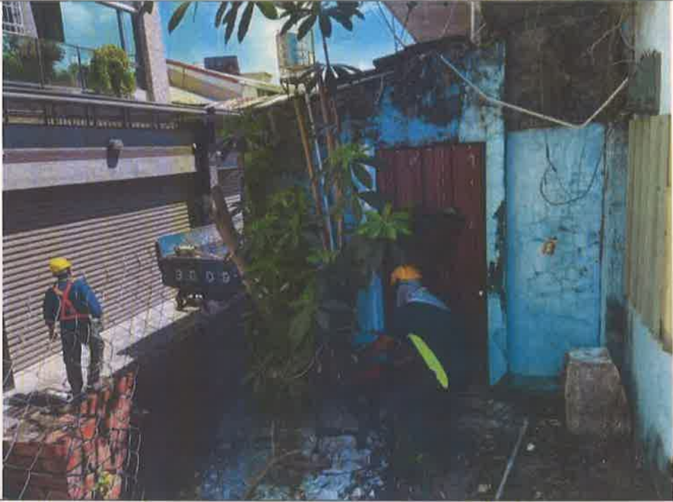
施工中照片1 Photos during construction1
