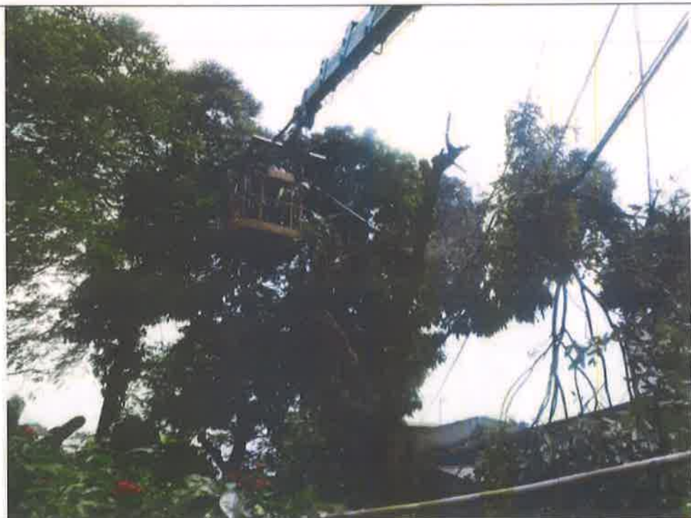
施工中照片2 Photos during construction2
