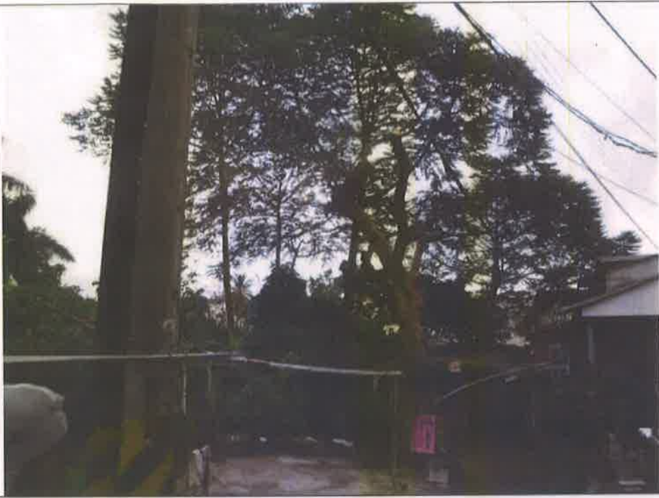
施工後照片1 Photos after construction1
