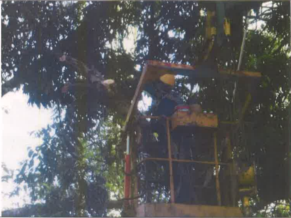
Photos during construction1
