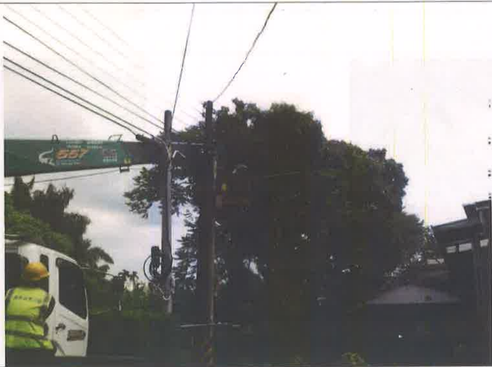
施工中照片1 Photos during construction1
