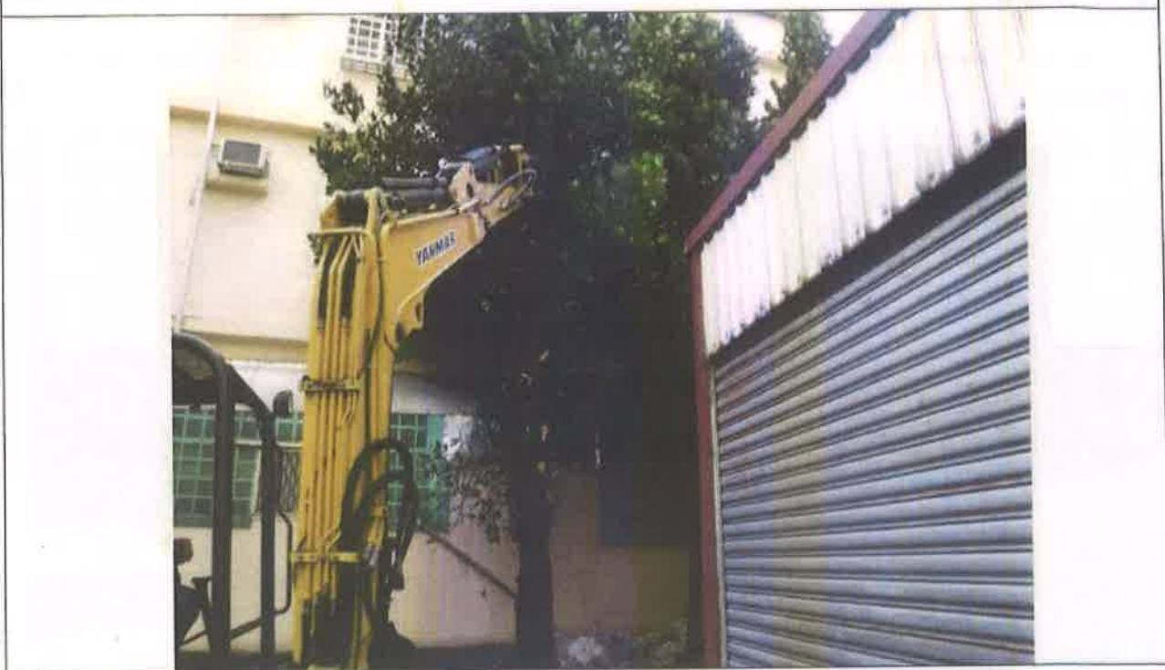
施工中照片1 Photos during construction1
