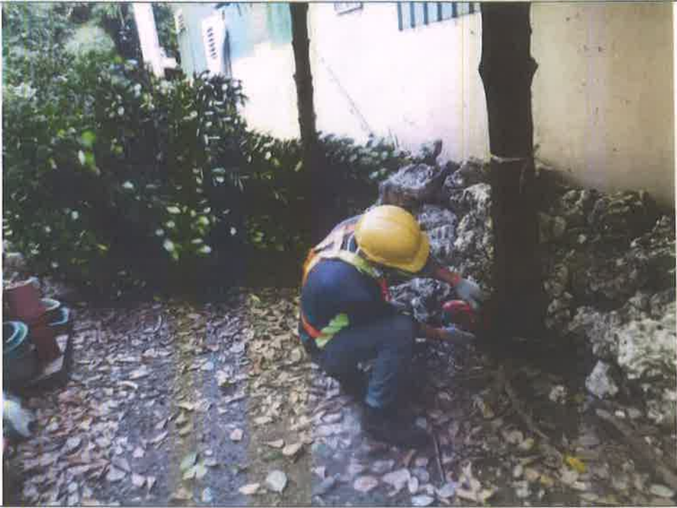
施工中照片1 Photos during construction1
