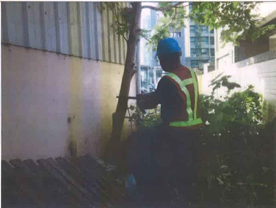
施工中照片2 Photos during construction2
