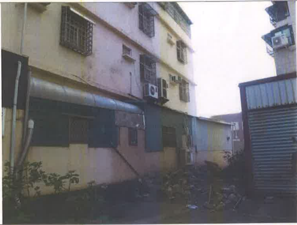
施工後照片1 Photos after construction1
