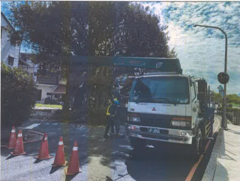
Photos during construction2
